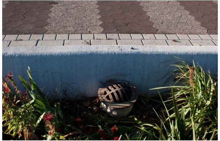
Figure 60 Storm drain planters
