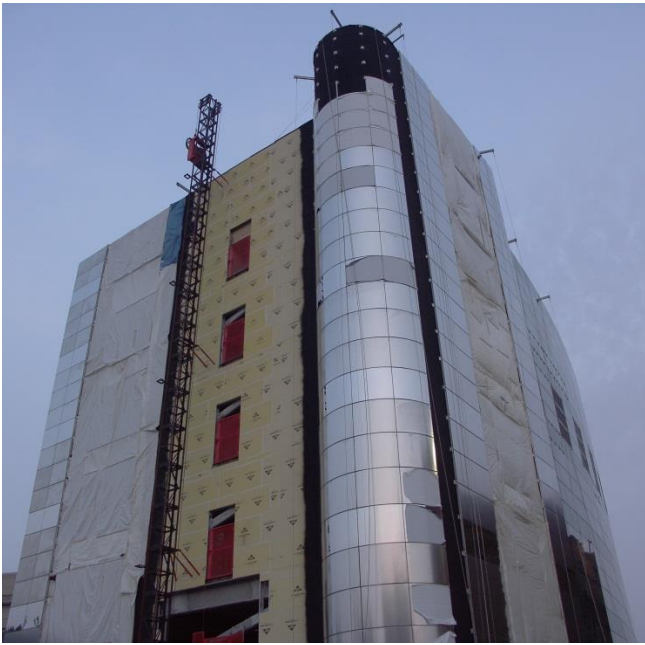
Figure 24 Installing steel outer wall
