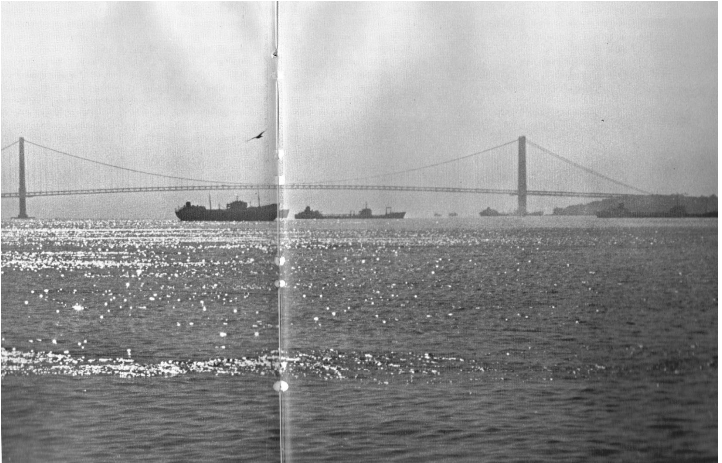
Figure 12 Verrazano Narrows Bridge
