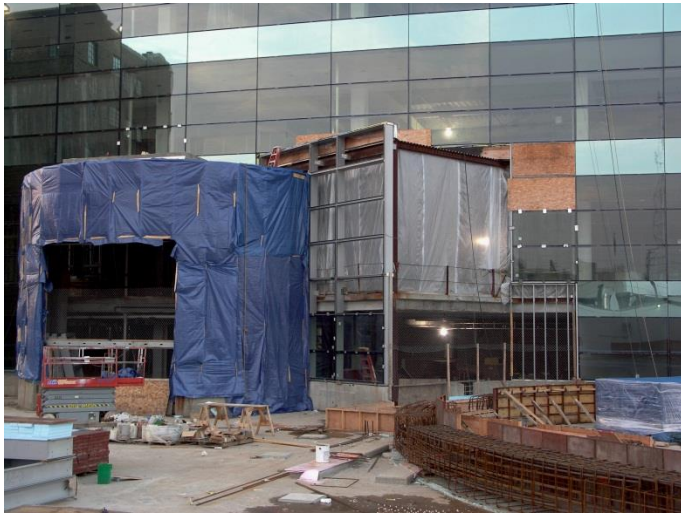
Figure 25 Installing glass walls
