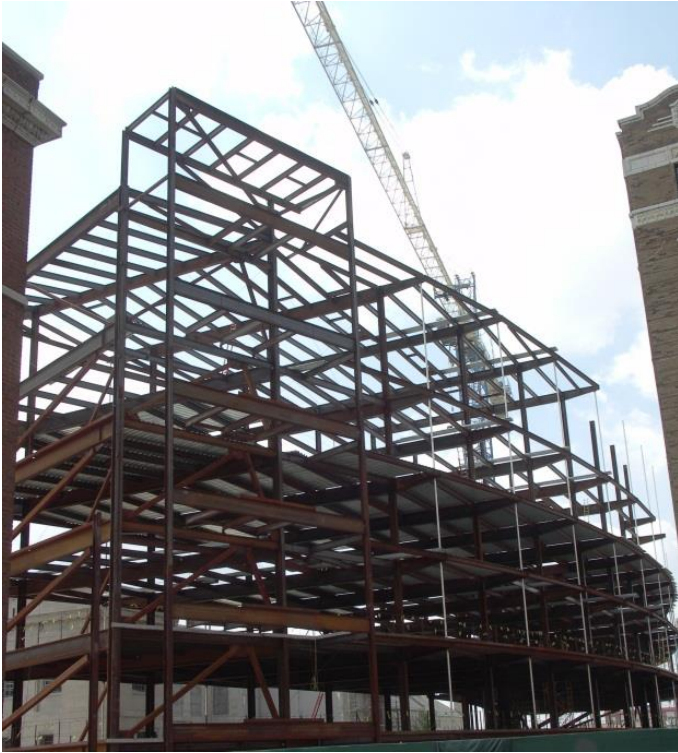
Figure 23 Library construction progress
