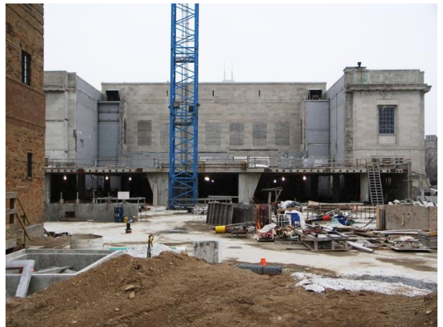
Figure 22 Library construction begins
